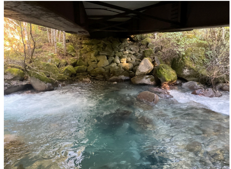
Left Bank Abutment when facing downstream
