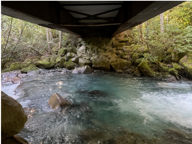
Right Bank Abutment when facing downstream
